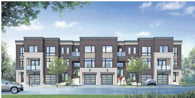
Frenchman's Bay, with its 57 three-storey townhouses and 10 detached two-storey dwellings, 'allows that end user from Toronto currently in a condo to move into a larger unit.' MADISON GROUP
